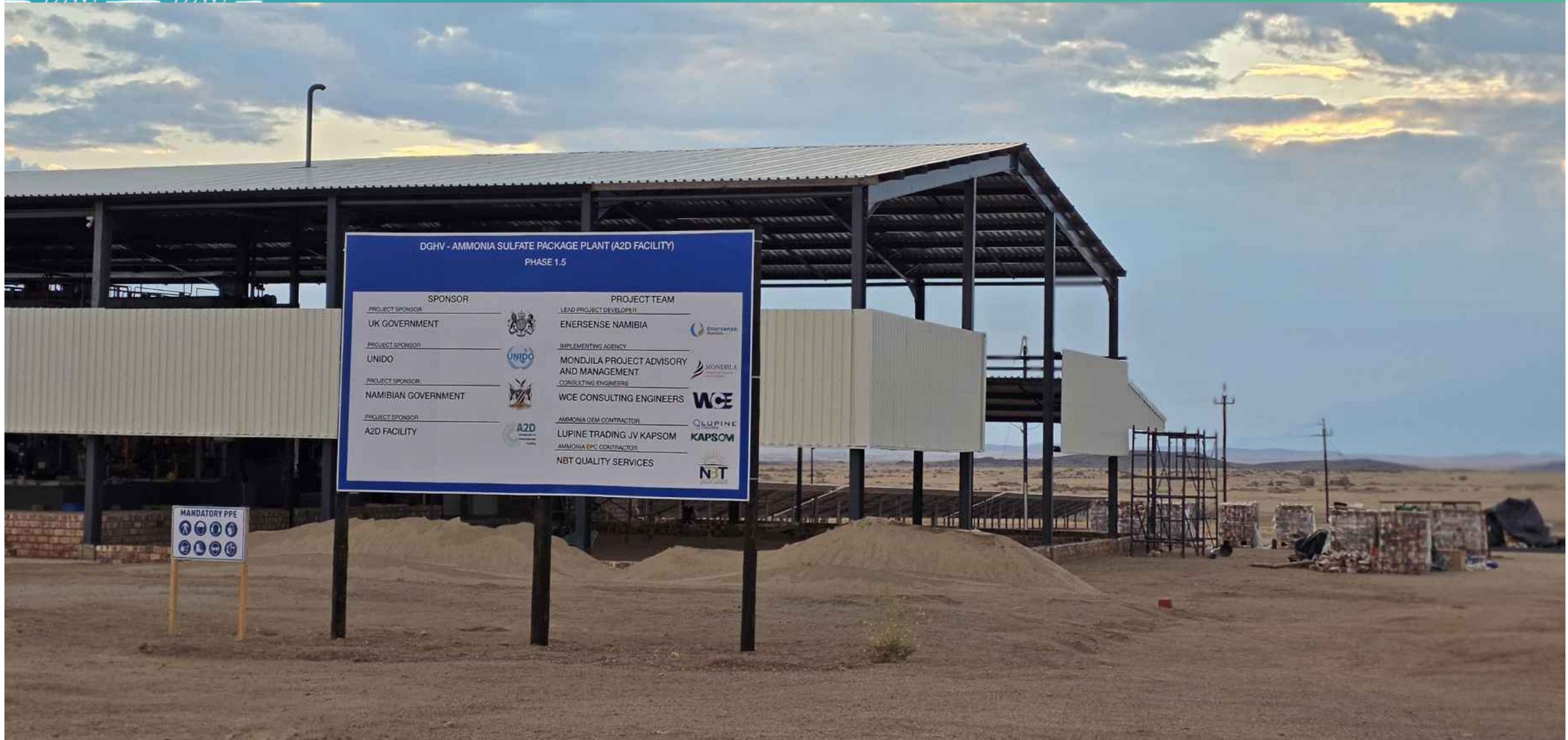
Above : Bulk earth works for the ammonia sulphate package plant now complete
