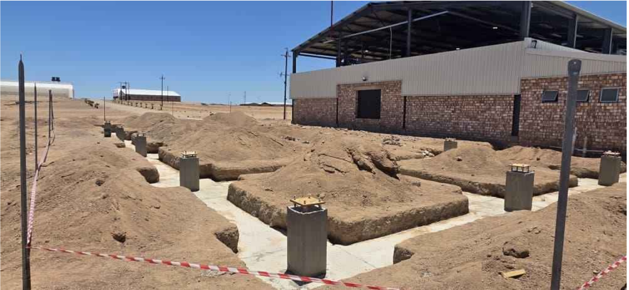
Above : Concrete works Completed
