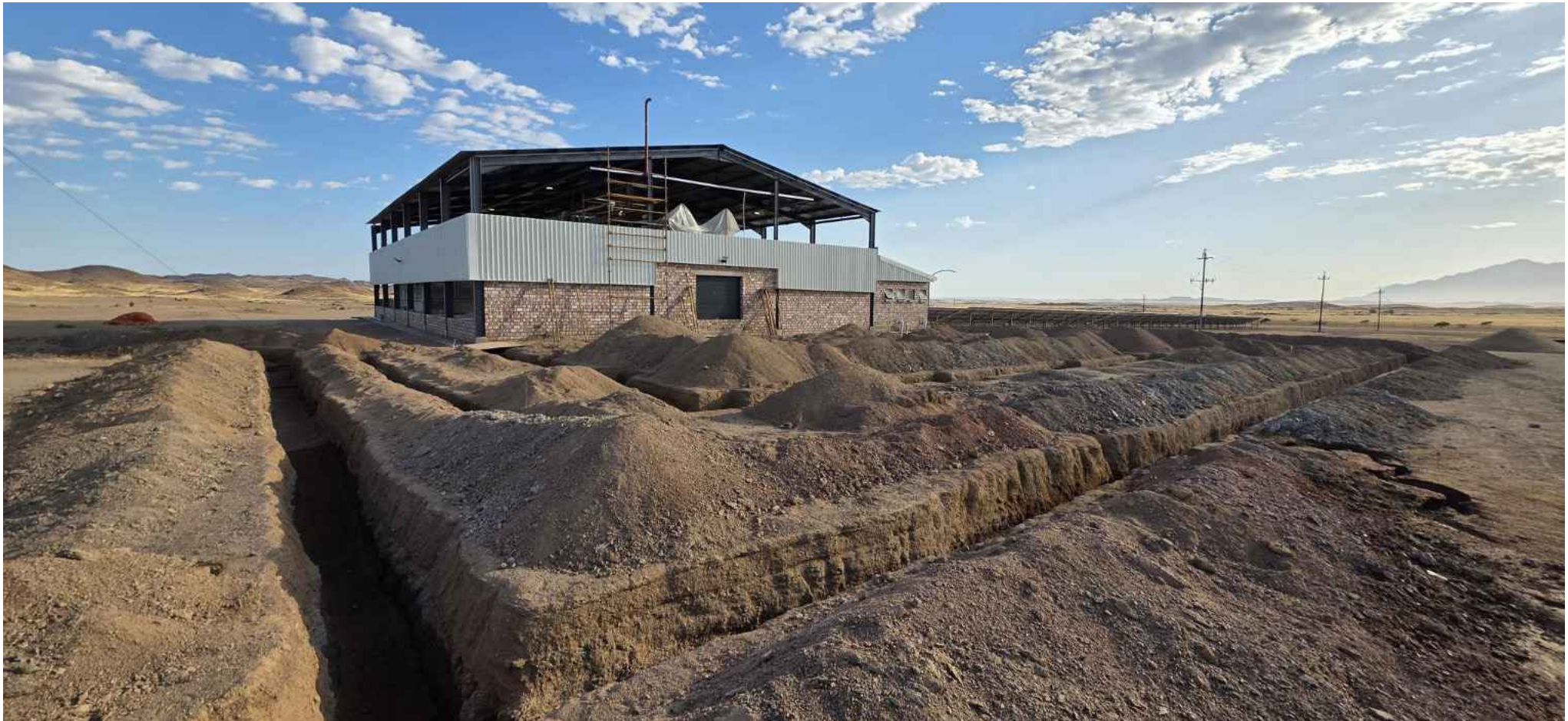
Above : Bulk earth works for the ammonia sulphate package plant now complete
